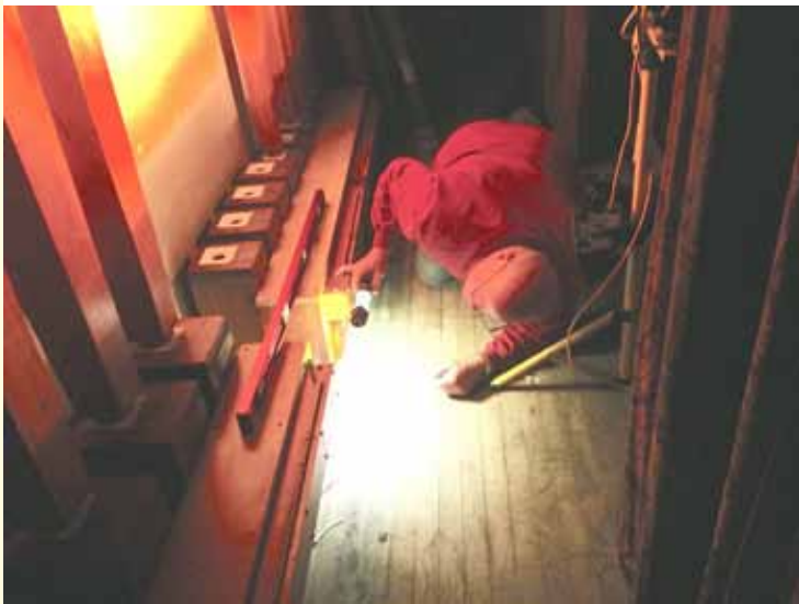
Bob MacNeur checks alignment of chests (photos: Jack Powers)
